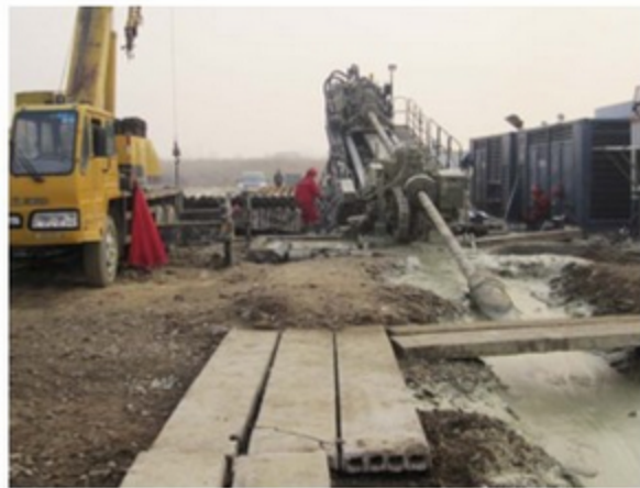
Prime Horizontal: An American Augers drilling rig.
