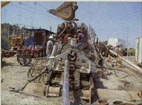
This project involved two intersects, each more than 7,300 ft.
