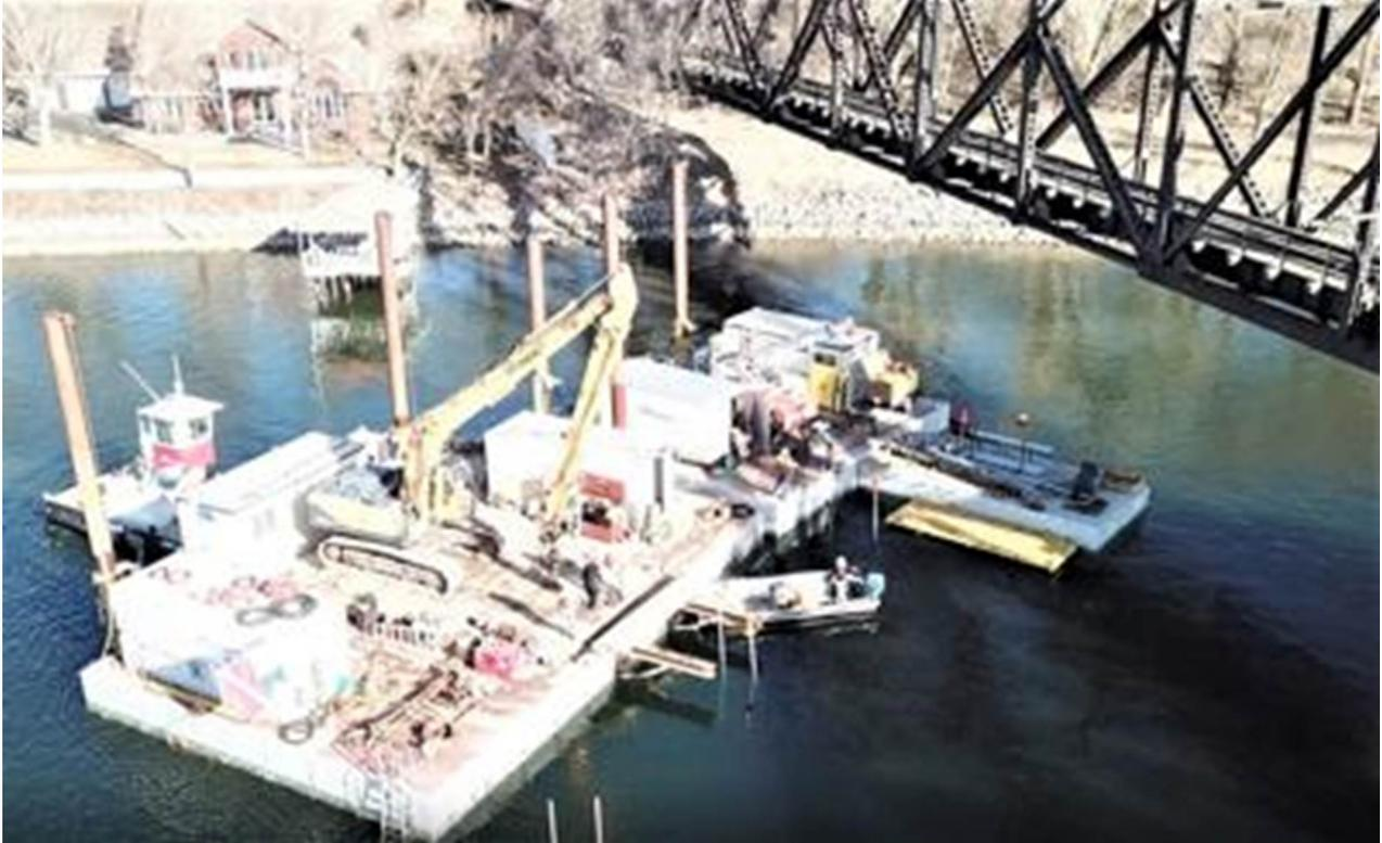
This floating platform is home base for underwater excavation and construction work for the drinking water treatment facility. The platform has an excavator, indoor office, four shipping containers, several docks, bathroom, other equipment, and a dozen people. – Photo provided by city of Pierre
