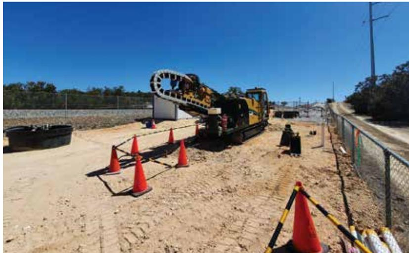
The job required the drilling of 2 crossings using jetting technique and steering with ParaTrack Gyro Module (PGM) which was a requirement from the project owner. Particular care and caution was taken as drilling was within 1m (at its closest point) of an existing gas pipeline, overhead power lines, railway tracks, as well as, other underground communication services lines posed a magnetic challenge.
