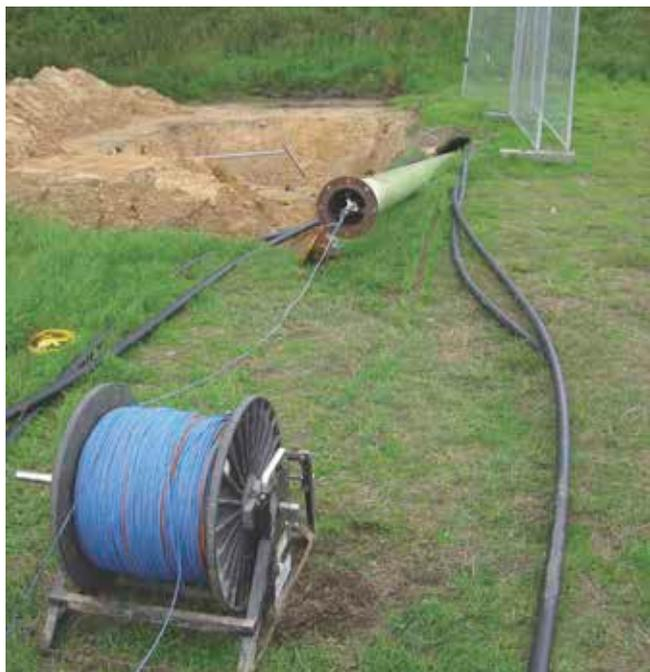
Figure 2. Data collection: the GyroTrack tool in the pipe
