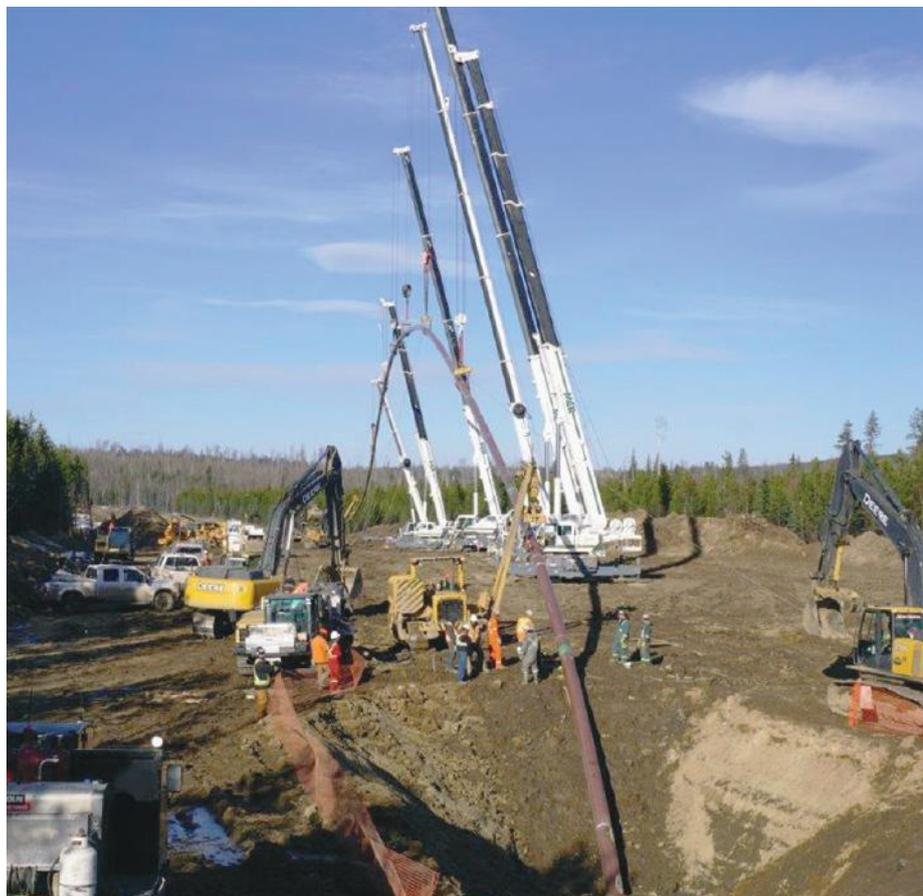
The Rig is in place and the centralizer casing is being lined up.
