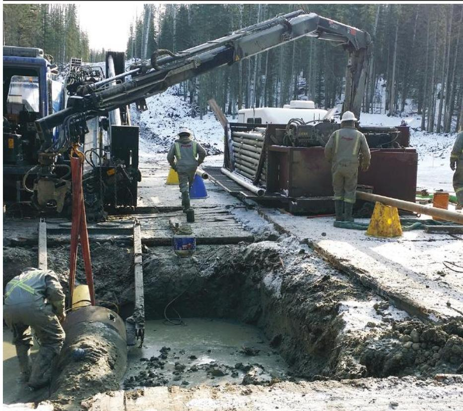
Results from the RMRS system can be well modeled with up to 40 meters of separation, where Passive Magnetic systems struggle beyond 4 meters. At close range the RMRS resolution is more enhanced, supplying operators with better data to make more accurate steering decisions. The rig on exit side was mobilized first and drilled 480m of the pilot hole, and then reamed
