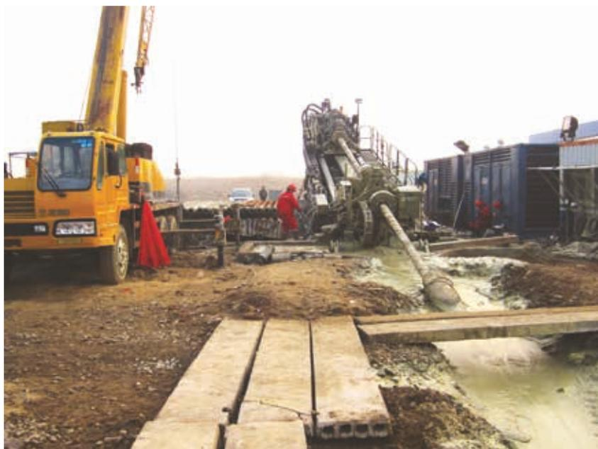
Figure 1. One of the American Augers drilling rigs.
