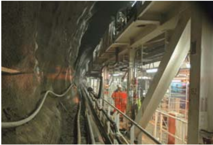
View down the 240 m-long mixshield TBM
